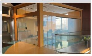
The natural light entering the room causes the PDLC film to have an increased haziness here when looking in from outside of the room. If it was dark outside the exterior windows the haziness would look different. Viewing from different angles also changes the appearance.
